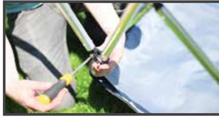
7. Attach rear support poles to the back using the black nylon brackets. Secure with provided nuts and screws.
